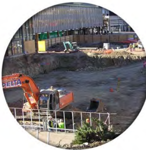
The Link groundwork
